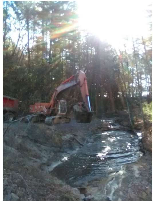
Image 1 - The work at Bedpost. This shot shows how carefully the dredger repairs the haul path and the sides of the trap as work is finished
