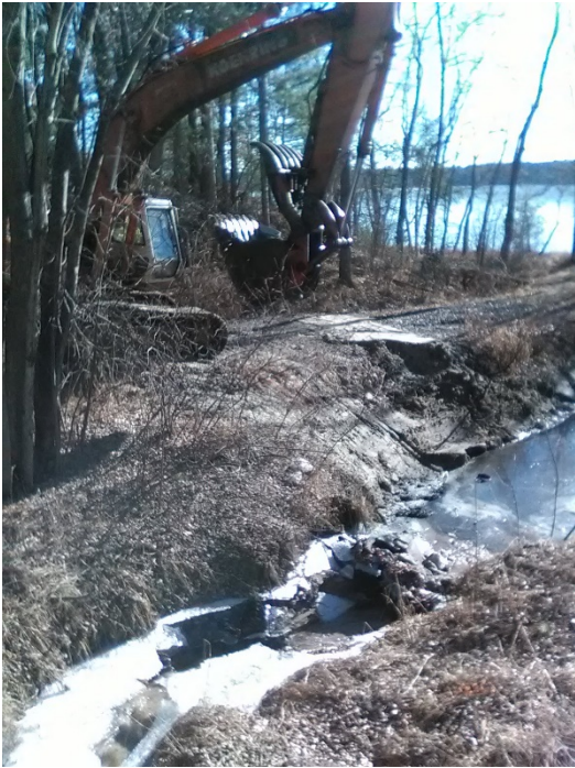
Image 1 - The work at Bedpost. This shot shows how carefully the dredger repairs the haul path and the sides of the trap as work is finished
